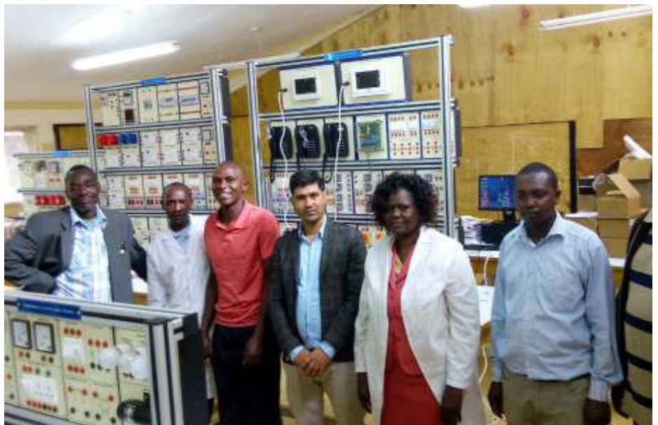
Installation at Eldoret National Polytechnic, Kenya
